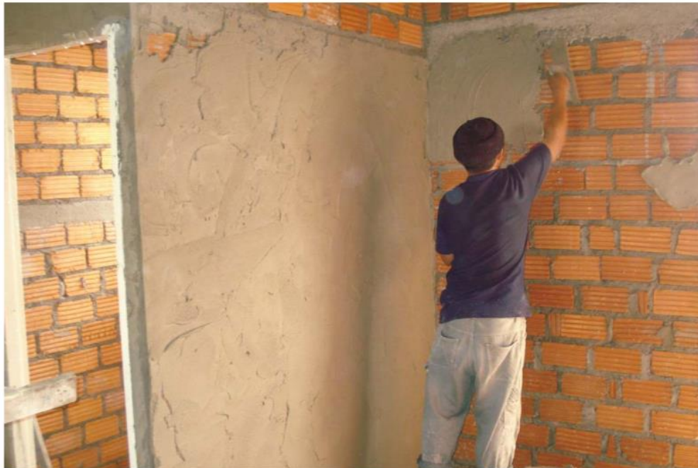
Figure 24: Plastering of brick walls (Thovichit, 2007)
